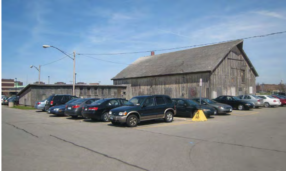
Building 30 – Wagon Shed
